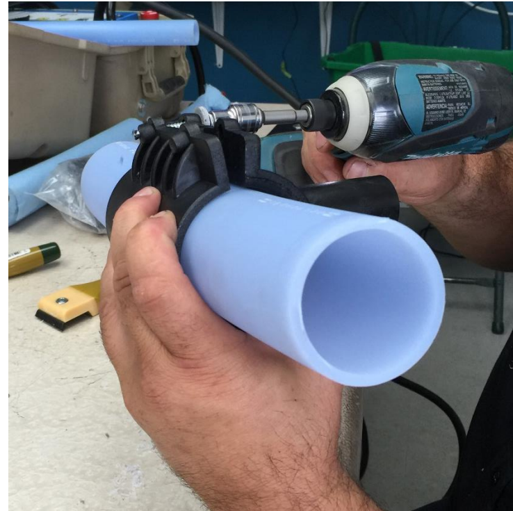
Install 2 screws on the opposite side, without tightening them completely, in order to be able to align the saddle with the hole on the pipe.
