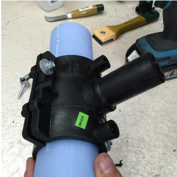
Install 2 screws tightly
