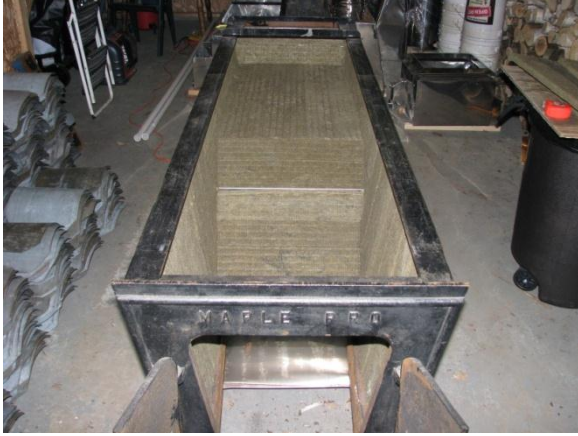
Insulation board laid out in the arch
