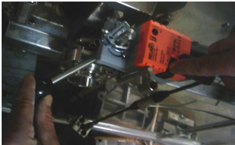
When you operate the thermoregulatory, at any moment, you can push the black button to free the valve. By releasing the button, the valve automatically returns to the right position.
