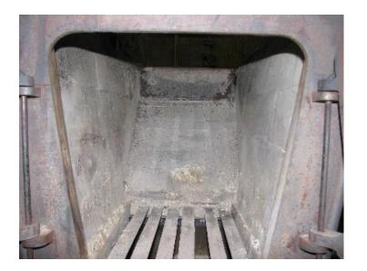
Final result. High temperature cement is used to hold the bricks together and seal the leaks.
