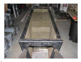
Insulating panels installed in the evaporator.
